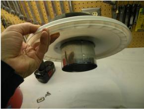
Take completed vent assembly and drop it into the 4-inch hole from the top of the lid. Mark, drill the 1/8 inch rivet holes in the lid and rivet together.
